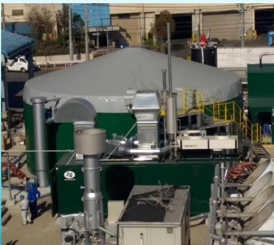
Built in 2015, this anaerobic digester runs on food waste only. It was designed to be very small because of its location in a crowded area. The Kishiwada plant exists to produce energy for the city of Osaka in Japan. Each year, 17 tons of food waste are converted to biogas and burned in a **co-generation** plant. The food waste comes from a waste processing facility that is nearby, so very little transportation is needed. This biodigester helps reduce the amount of waste produced by the city.
